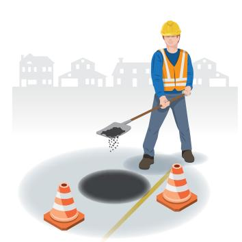
After the tack coat is applied the pot hole is filled with asphalt.
