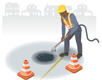
Next a tack coat is applied to the pothole to allow asphalt to stay in the pothole better.
