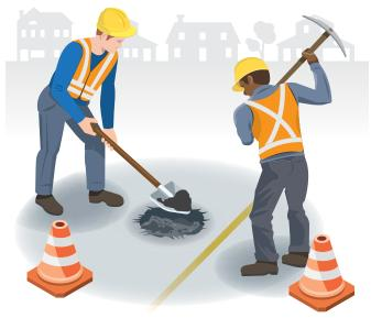
Then City crews remove any loose material, debris and water from the pothole. This is done using equipment like shovels and picks to remove debris and a torch to remove water.
