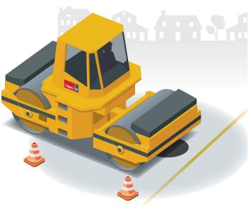
Once the pothole is filled it is compacted using a roller. The asphalt is compacted until it is level with the roadway.
