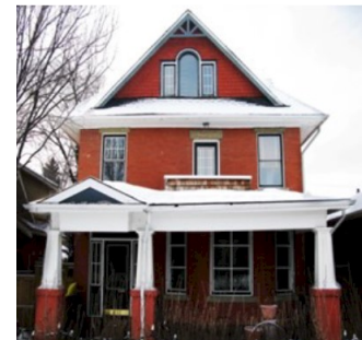
Robert and Mary Taylor Residence (built 1912) Designated Municipal Historic Resource
