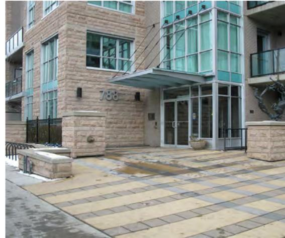
The two-coloured concrete paving material is used to accent the residential building entrance while coordinating with the textures of both the building facade material and adjacent sidewalk surface material.
