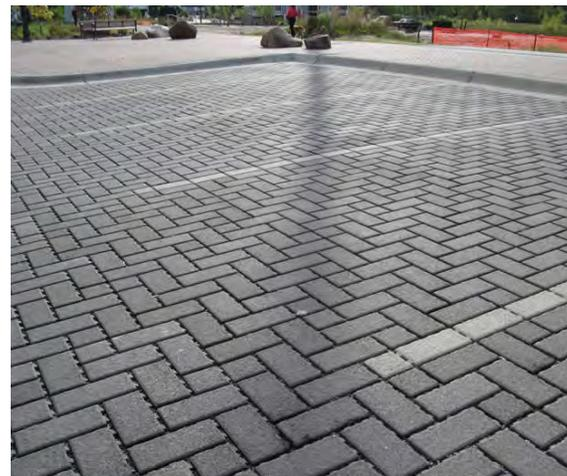
Permeable paving can be used to provide increased stormwater infiltration and minimize runoff.
