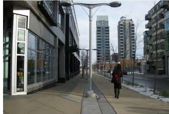
Pedestrian scaled street lighting along 13 Ave. Heritage Greenway.
