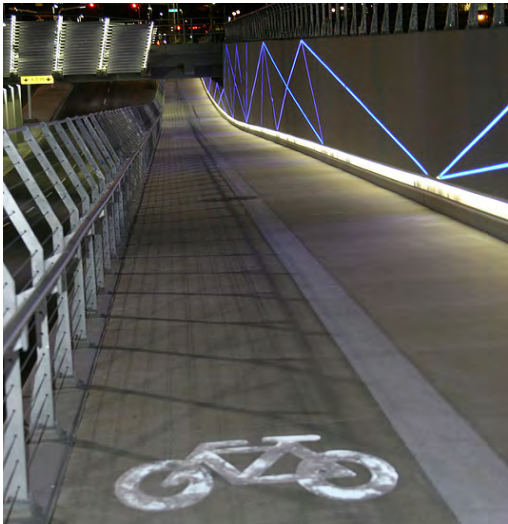
Multi-use pathway at 4 Street Underpass, Calgary.
