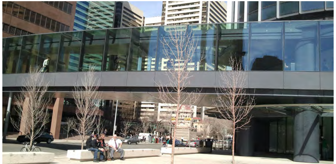
+15 Skywalk System linked to an at-grade sunny plaza.
