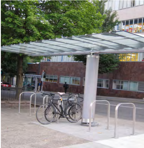
Covered bike parking, Portland.
