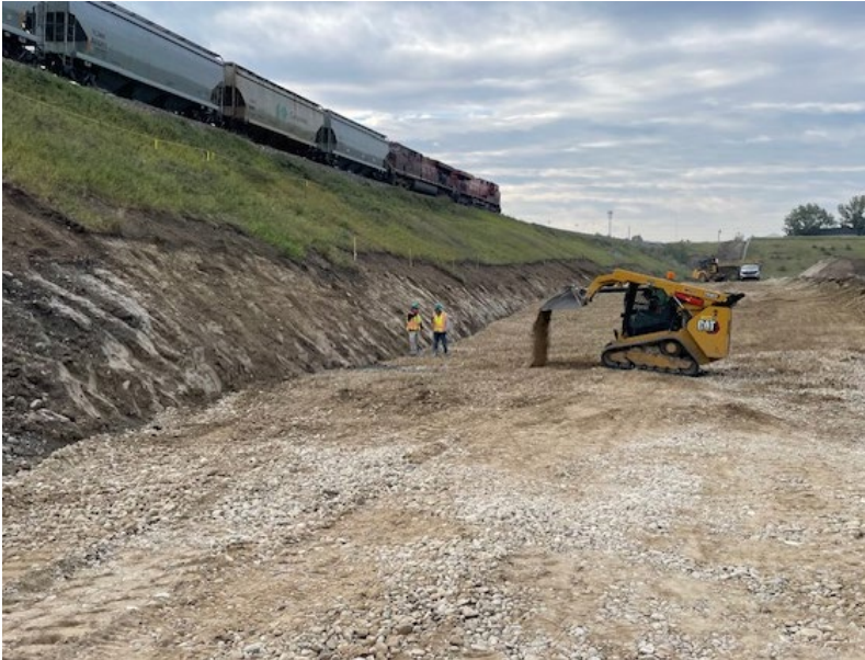
Looking south along the diversion track alignment.
