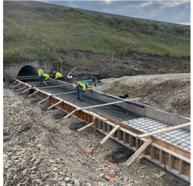
Looking east at the culvert extension
