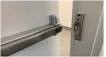
Strike plate allowing the door to mechanically override the lock
